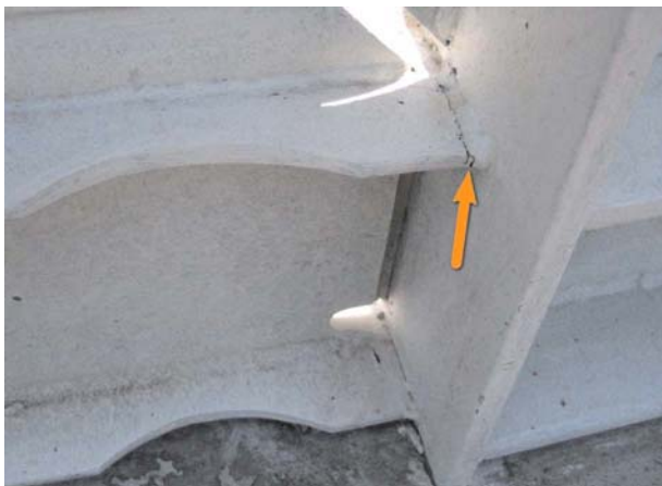
Fig. 11. Photograph of SPSW 1 bottom beam flange fracture
